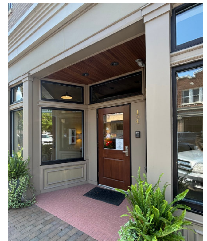
Building Facade Maintaining Earth Colored Tones in Downtown Florence
