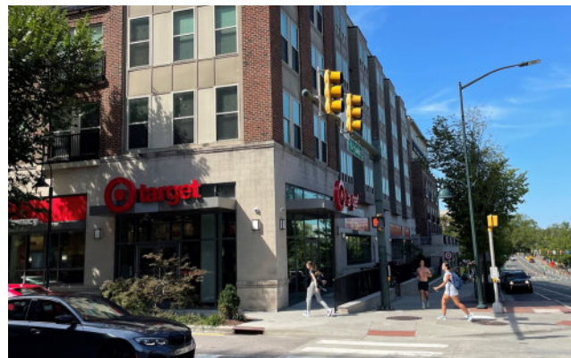
Modified Franchise Design Integrated into the Ground Floor in Chapel Hill, NC
