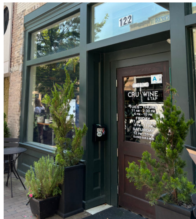
New Wood Door and Refurbished Windows in Downtown Florence
