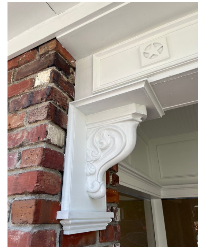
Preserved Cornice On A Downtown Florence Storefront
