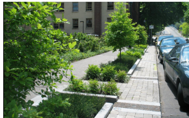
Bioretention Planting Strip | City of Portland, OR
