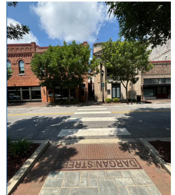
ADA Pedestrian Crossing on North Dargan Street
