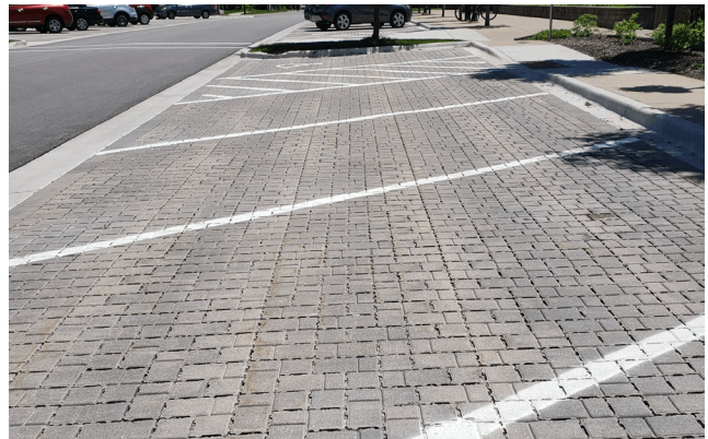
Pervious Parking Paving | City of Warrenville, Illinois
