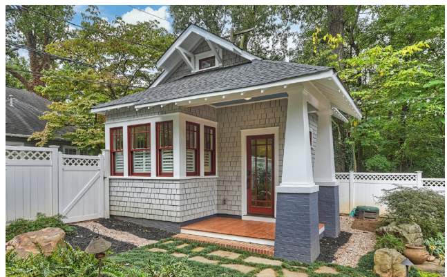
Complementary Accessory Structure | Hopedale Builders
