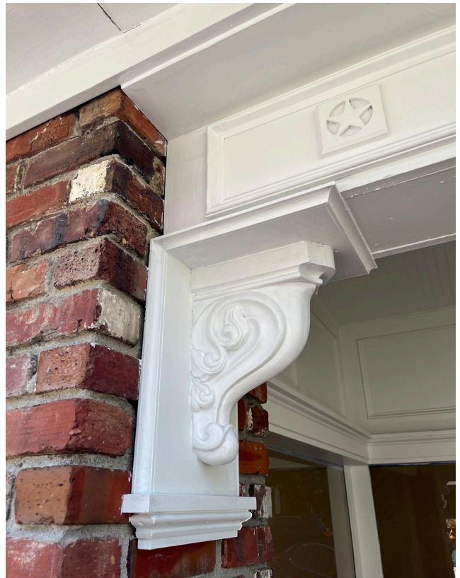
Preserved Cornice On A Downtown Florence Storefront
