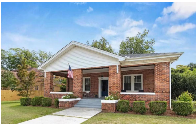
Home With Brick Foundation and Porch in Timrod Park | Homes
