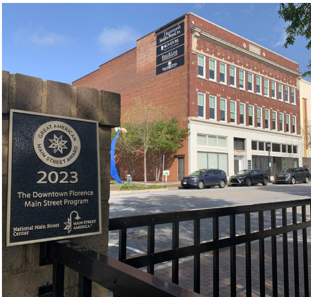
Rehabilitated Historic Waters Building | Municipal Association of South Carolina
