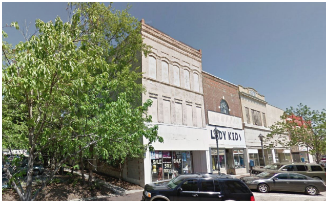
127 West Evans Street Renovation Before | Google Earth
