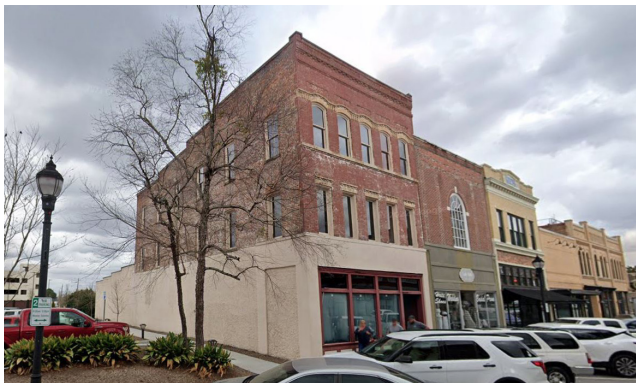
127 West Evans Street Renovation After | Google Earth
