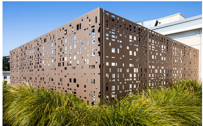
Mechanical Equipment Screening | BOK Modern
