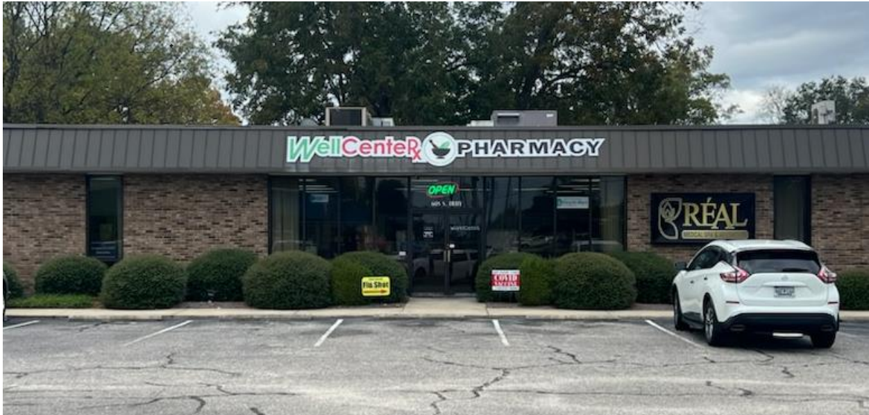
East side facing South Irby Street.
