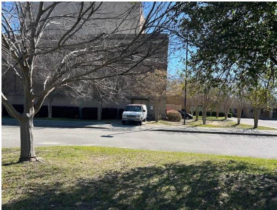
East view facing the storage building.
