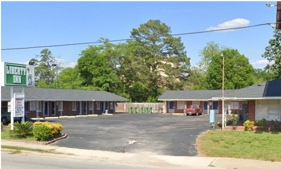
View of the fence between the back of Liberty Inn and proposed site
