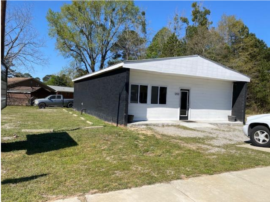
Existing commercial building on north side of lot.
