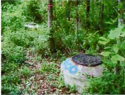
Manholes Along Southern Interceptor
