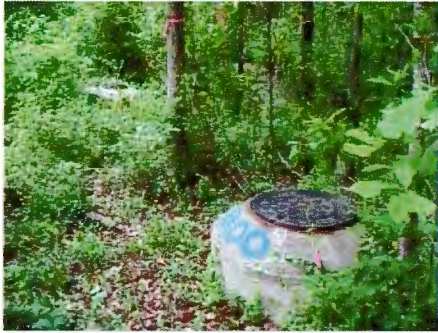
Manholes Along Southern Interceptor
