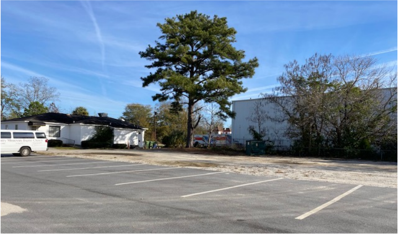
Rear of house at 212 West Sumter Street (youth building) and east property line.
