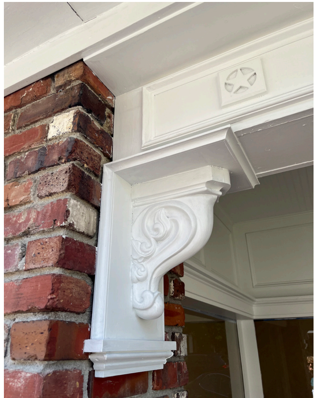
Preserved Cornice On A Downtown Florence Storefront
