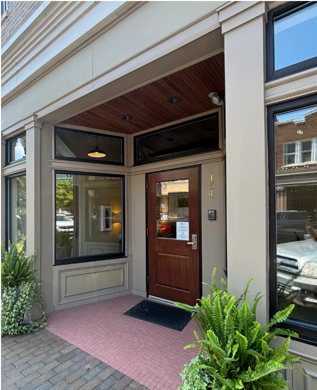
Building Facade Maintaining Earth Colored Tones in Downtown Florence
