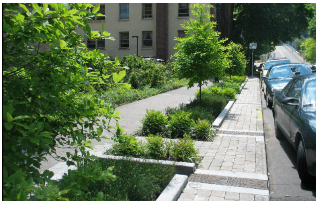
Bioretention Planting Strip | City of Portland, OR
