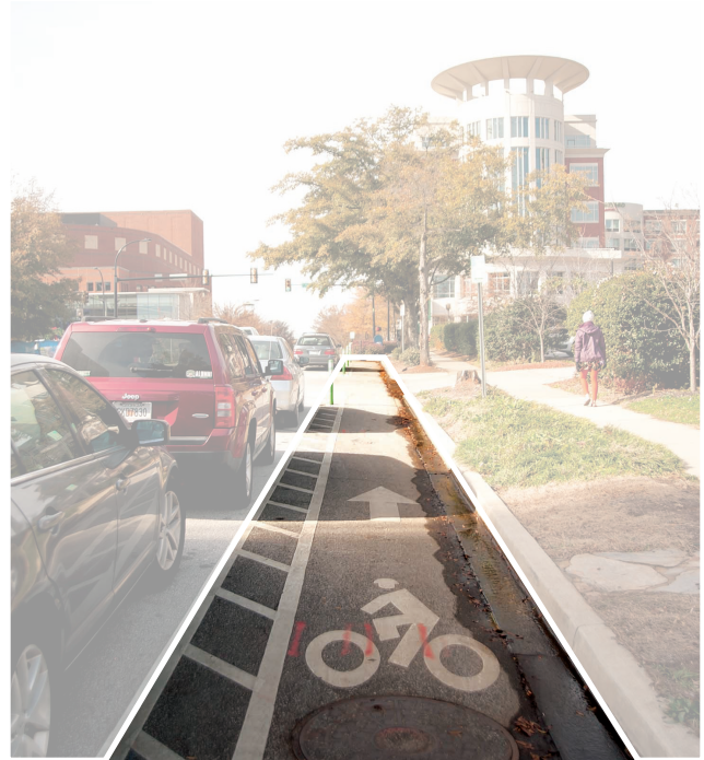
Bicycle Lane in Greenville, SC | Michael Dantler
