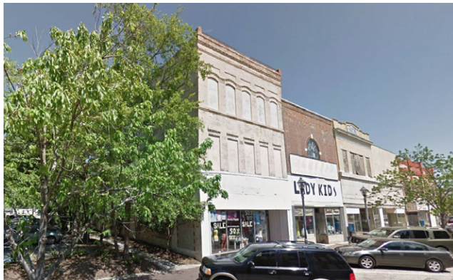
127 West Evans Street Renovation Before | Google Earth
