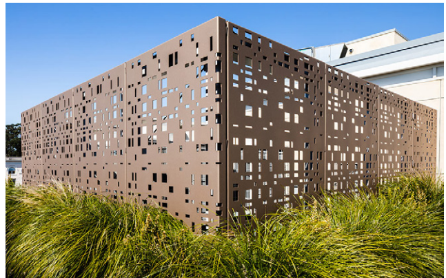
Mechanical Equipment Screening | BOK Modern
