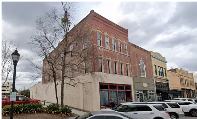
127 West Evans Street Renovation After | Google Earth
