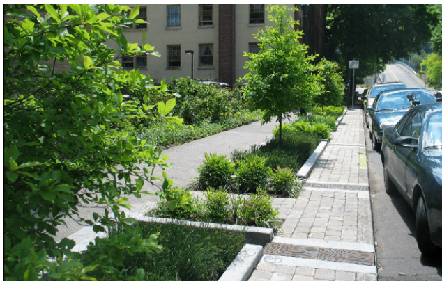
Bioretention Planting Strip | City of Portland, OR
