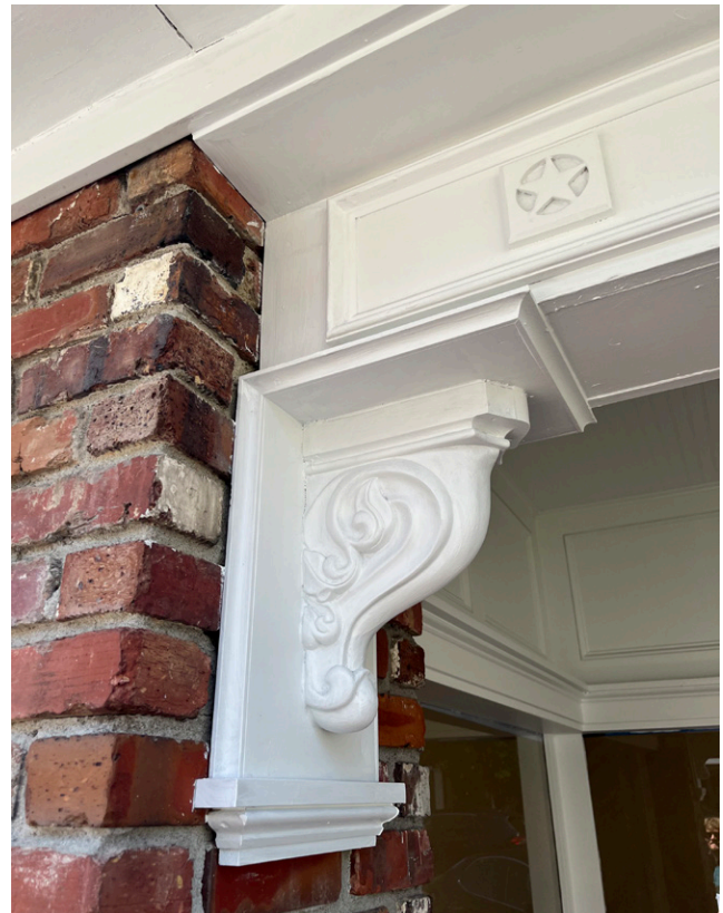
Preserved Cornice On A Downtown Florence Storefront
