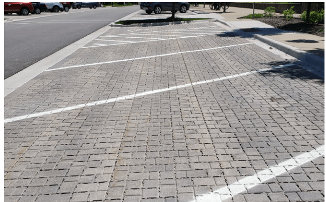
Pervious Parking Paving | City of Warrenville, Illinois
